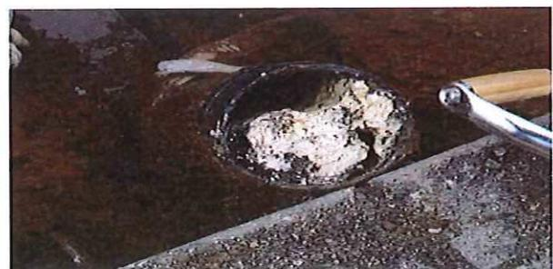
This is a 6 inch house sewer. Over 90% of this lateral was blocked by grease accumulation. This caused a back-up in the residence and cost \$3,800.00 to repair.
